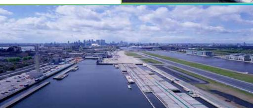
This view overlooking the docks, towards the city, captures the new deck structure that is under construction adjacent to the existing runway. Eight new aircraft stands will sit on the deck, as well and the terminal areas, including departure lounges. Also on the left side of the photo, the new Digital Air Traffic Control Tower is visible that will enter operation early next year.
