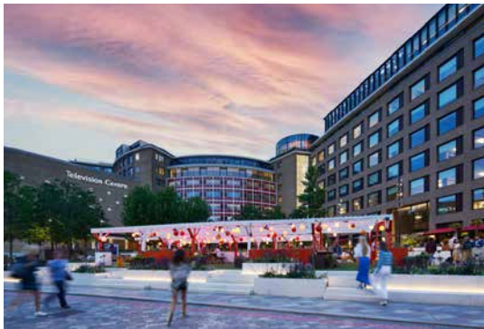
Solar at Pergola, Television Centre
