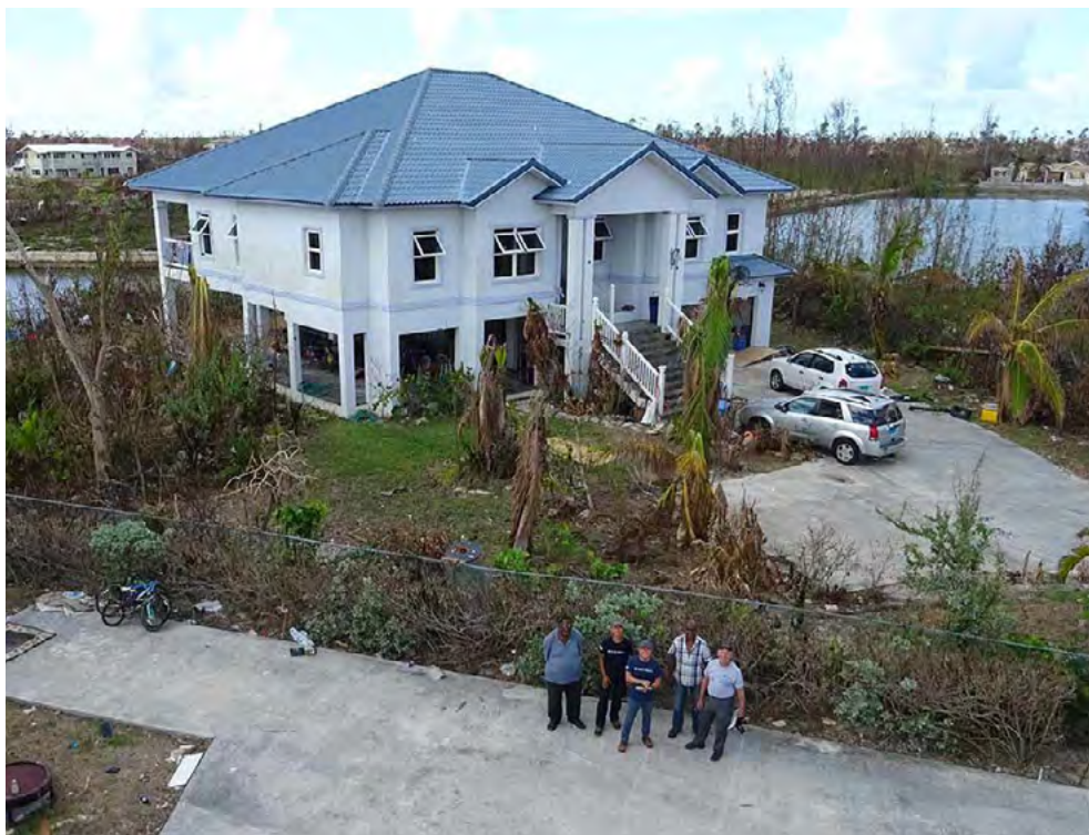
The construction of this home allowed it to survive Hurricane Dorian. The neighbor's homes were destroyed
