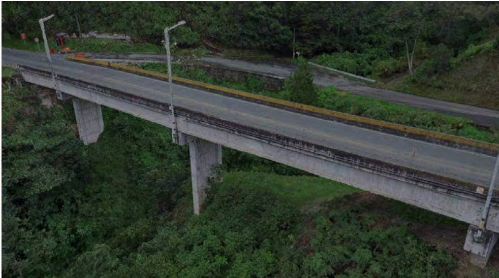
3D rendering of the bridge that was renovated in Autopista al Mar 1 road in Colombia
