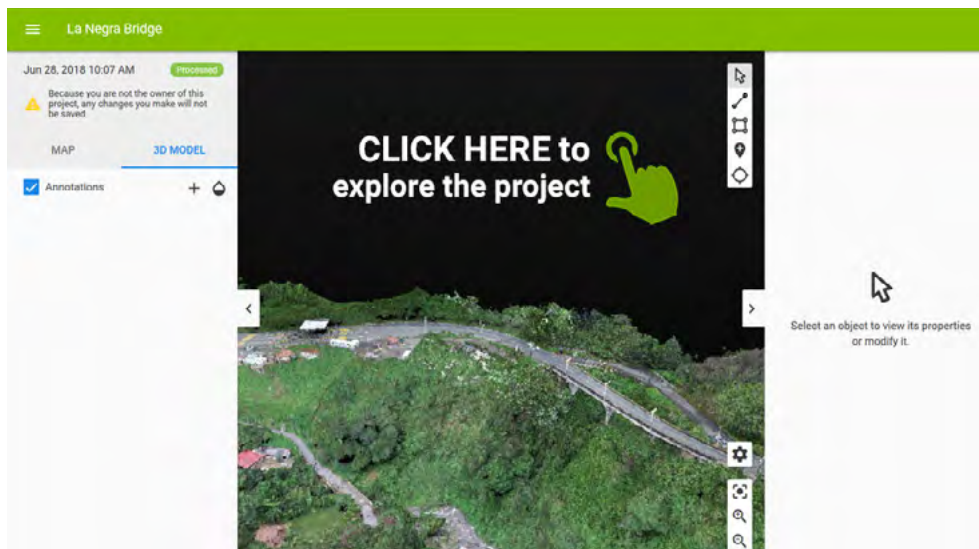
Click on the image to explore the 3D render of La Negra Bridge
