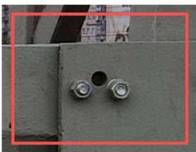
Annotation 2 Annotation type: To be fixed Severity level: 5 **Description:** Missing bolt
