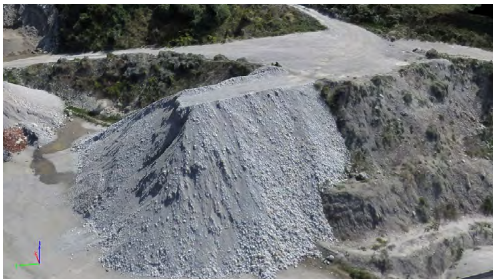
Ramp stockpiles can store large amounts of material. Data set source: courtesy of Geomatic Development
