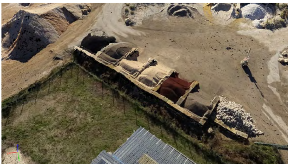
A bin stockpile is surrounded on three sides, enclosing the material. Data set source: courtesy of Geomatic Development
