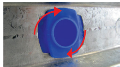
Attachment of the dowel sleeve
