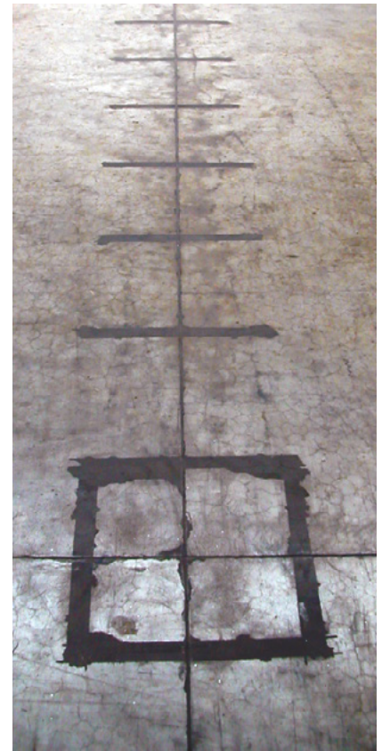
Refurbished saw cut joint with supplementary dowel bars
