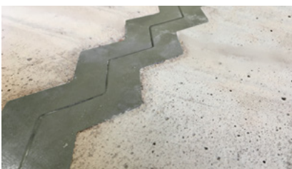
Joint after concreting
