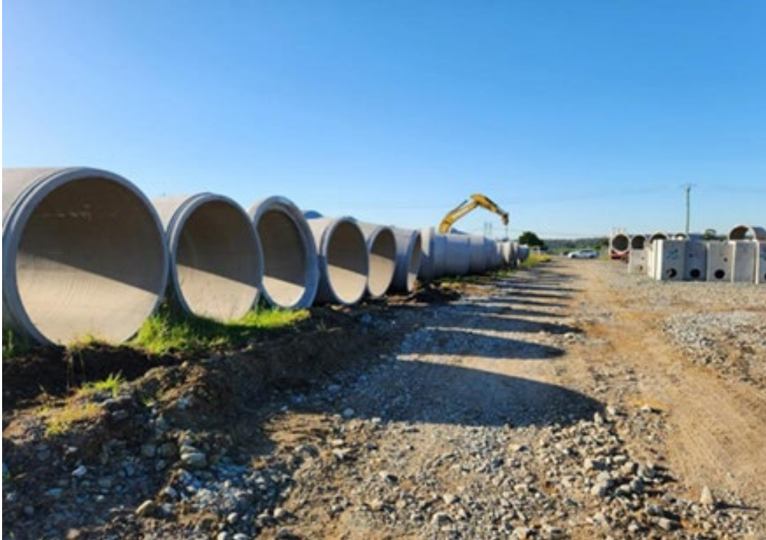
Summerset's Cranbourne North site under construction
