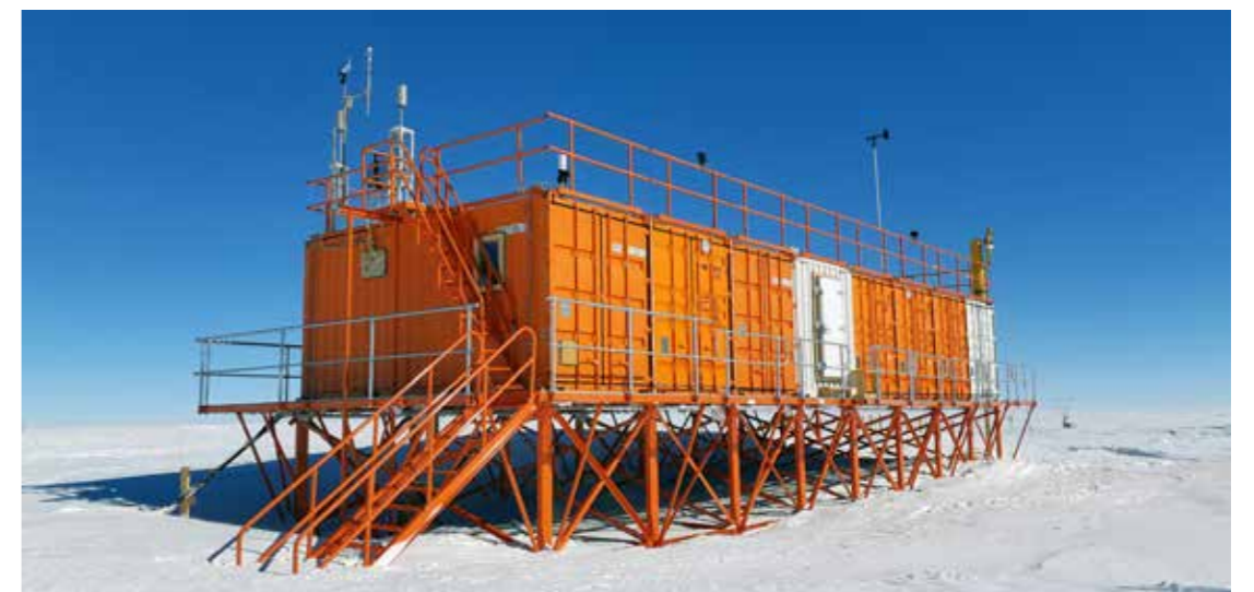
Concordian puhdistilalaboratorio mittalaitteineen. The clean air facility at Concordia housing the measurement equipment.
