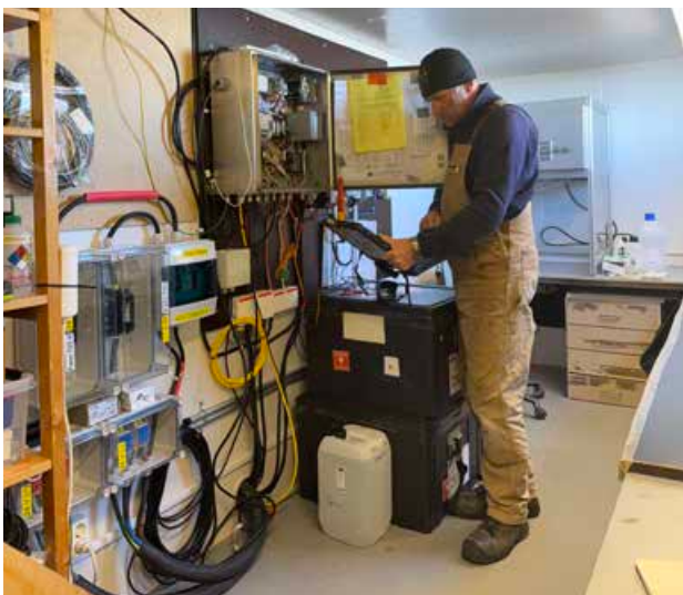
Priit Tisler servicing the research station’s automatic weather station.
