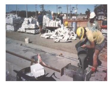
TamCrete HF is a non-shrink, cement based, which is specially formulated for use in critical grouting operations where positive expansion and non-staining characteristics are required. A high strength free flowing cementitious grout based on non-reactive aggregate, low alkaline shrinkage compensated Portland Cements with selected admixtures which produce a chloride-free grout. TamCrete HF contains a maximum size aggregate of 2 mm and is suitable for grouting thickness of between 5 mm and 75 mm.
