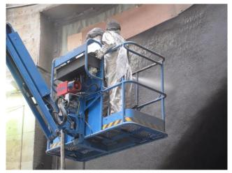
TamCrete TopShot is a specially formulated cement based, pre-bagged, gunite mix for dry spray application. It is suitable for sprayed repairs, infilling of piles and is designed to be used as a regulating layer in sprayed concrete linings. TamCrete TopShot can be supplied with the inclusion of microsynthetic fibres to provide fire resistance properties.
