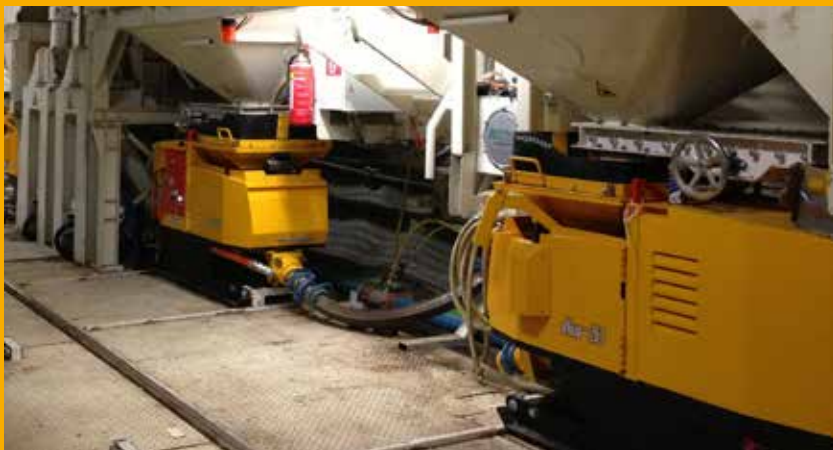
Pea gravel backfilling installation on TBM
