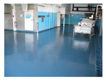
TamRez 530 is a two-component water-based coating. It is a low odour, epoxy-polymide coating. TamRez 530 is a high performance floor coating system designed to provide excellent wear resistance in combination with protection against chemical attack for concrete surfaces. It can be applied to new, cured or old concrete.
