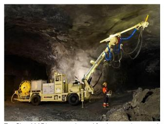
TamShot 90AF is commonly used for the wet mix sprayed concrete processes in the tunnelling and mining industry. The product is applied where initial ground support is needed or where a permanent lining has been designed (such as for single shell tunnel lining).
