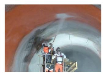
TamSeal 800 is a high performance, single component EVA polymer, flexible waterproofing membrane. Its typical use is for the waterproofing of sprayed concrete lining applications, where TamSeal 800 is spray applied using a dry rotor pump and sprayed by hand or robotic manipulator. TamSeal 800 provides a tough, durable, seamless, waterproofing membrane for many structures including tunnels, shafts, caverns and below grade box structures.
