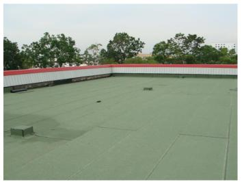
TamSeal 4000E is a 4.5 kg APP modified torch-applied bituminous waterproofing membrane. The surface is mineral slate, coated on a heavy duty high strength, non-woven polyester mat. The mineral slate provides excellent UV protection and is suitable for light pedestrian traffic. The rigid nature coupled with excellent UV resistance of the membrane provides for long weathering and maintains the properties for an extended period of time.
