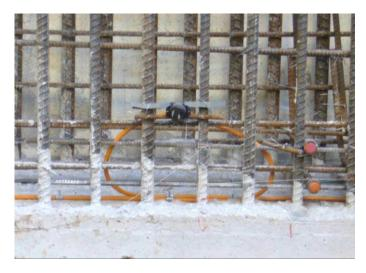
The Normet Injection Tube system is essential for the construction of water tight structures. The joints should be arranged in such a way that crack formation is virtually eliminated.
