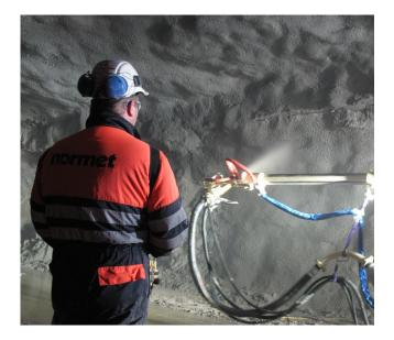
TamCem iBond is an aqueous, solvent-free, chloride-free internal curing agent designed for wet-mix sprayed concrete to improve the bond between the sprayed concrete layers and/or to the substrate, and to reduce rapid evaporation of water from the sprayed concrete, typically in permanent sprayed concrete tunnel linings exposed to high levels of ventilation draught, or low relative humidity.
