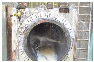
TamPur 120 is based on a polyol component (part A) and a polymeric MDI (part B). When mixed, a hydrophobic polyurethane is formed which is tough, rigid and resistant to a wide range of chemicals. TamPur 120 fast set reacts rapidly enabling the product to cut off large water leaks. TamPur 120 slow set has a long open time allowing for greater penetration into fine void and fissures.
