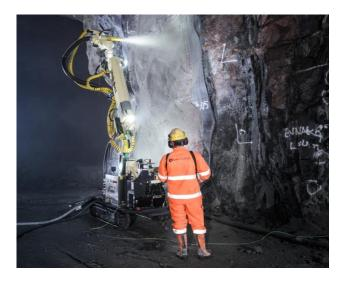
TamCem NanoSilica is a pozzolanic alternative to traditional cementitious replacements for durable concrete that provides sulphate resistance equivalent to typical microsilica (silica fume) at a much reduced dose. TamCem NanoSilica is used in wet mix sprayed concrete processes for tunnelling and mining applications.
