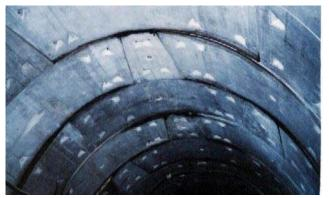
TamCrete TP is a shrinkage compensated, single-pack, cement based pointing mortar for use in areas where movement is anticipated. TamCrete TP exhibits good adhesion to cast iron, concrete blocks and concrete, making it suitable as a replacement for standard mortars where they have already deteriorated due to chemical attack or movement cracks.
