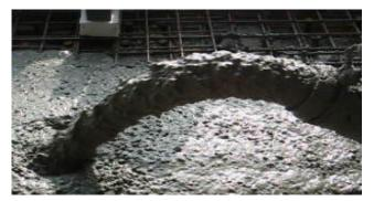
TamCem 77TG is a special "consistence modifier" for concrete and grouts with no water reducing effect, air entrainment or retardation properties. It is a non-chloride liquid admixture designed to increase pumping efficiency, reduce segregation, and enhances the viscosity and stability of high slump mixes.
