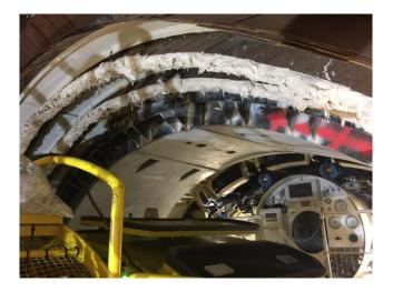
TamSeal TG92 is formulated as a first fill grade tail sealant to be used on shielded tunnel boring machines (TBM). Together with the wire brushes, the sealant forms an impermeable barrier between the tail shield of the TBM and the concrete segments to effectively seal off any ingress of water, soil and annulus grout/mortar back into the TBM invert.
