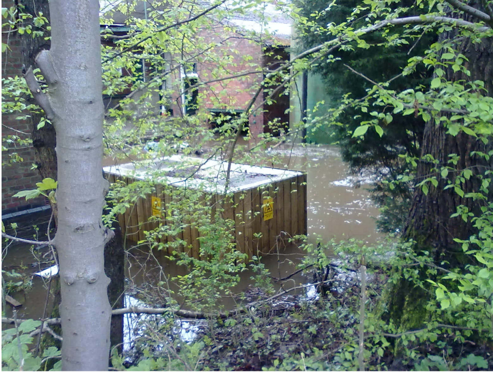
Figure 3: Flooding photograph (Source: member of public)
