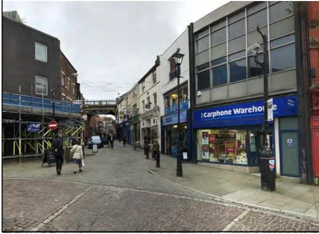
Inserted 1960's curtain wall in 19 th century building
