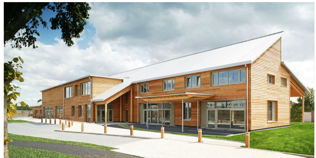
Oak Meadow Primary School in Wolverhampton built in 2012 to a space heating demand of less than 15 kWh/m 2 /yr (© Architype)
