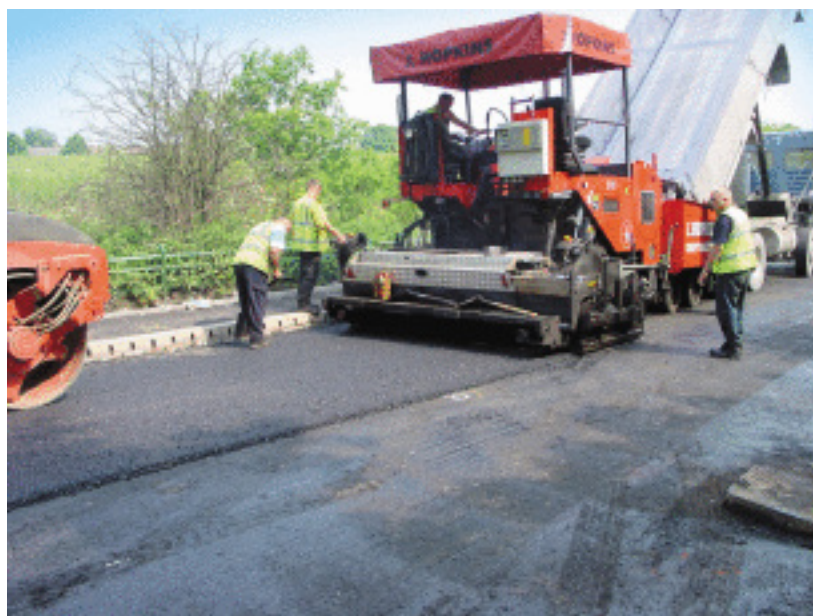
Picture 6.1 Carriageway Maintenance Works, Salford
