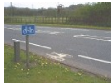
Picture 4.13 Cycle counter site, Rochdale
