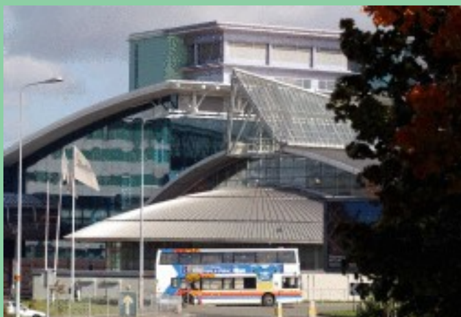
Picture 5.7 The Station, Manchester Airport
