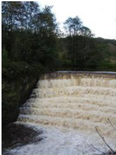
The stepped weir at the head of the river
