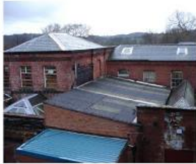
Engine House and Warehouse from Roadside Shed
