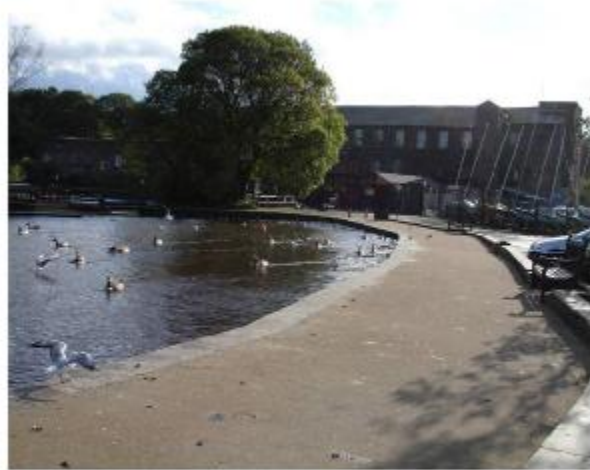
An area of infilled land exists to the north west of the reservoir forming a carpark
