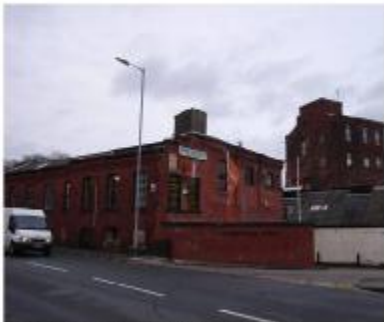
Engine House and Warehouse from entrance
