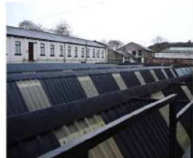
Large Weaving Shed
