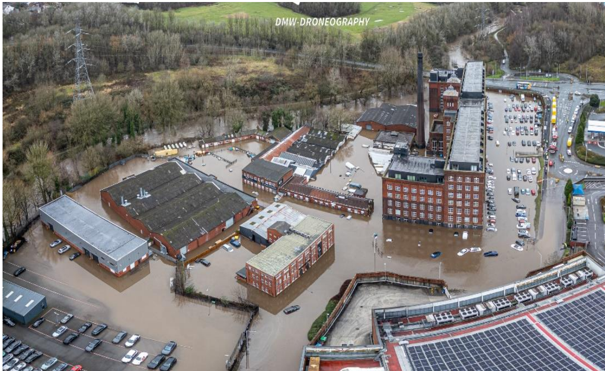
Figure A7.4. Image showing flood waters around Meadow Mill on 01.01.2025. Image Source: DMW Droneography (Facebook).
