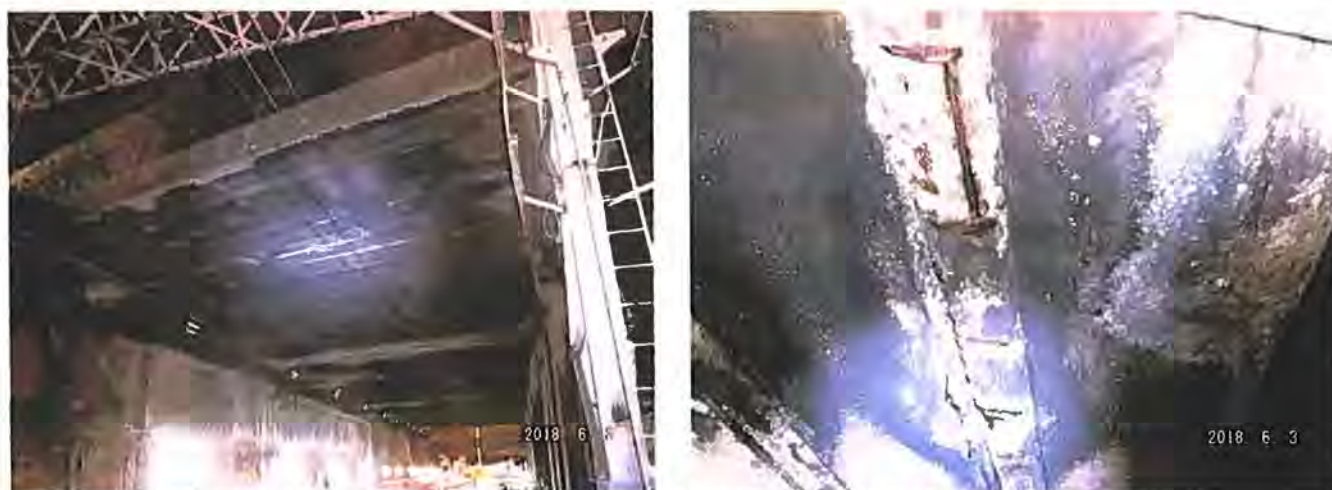
Figure 2: General view of the bridge and spalling to the deck of span 1, with exposed rebar.
