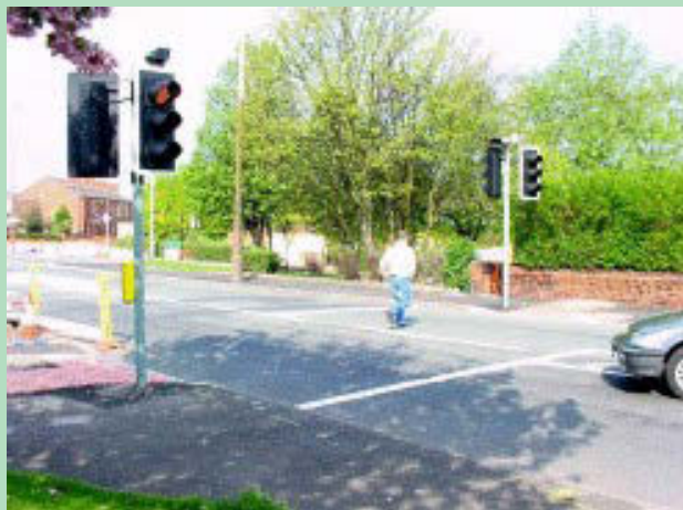
Picture 5.6 New pedestrian crossing, Tameside
