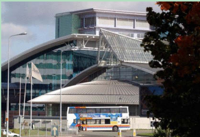
Picture 5.16 The Station
