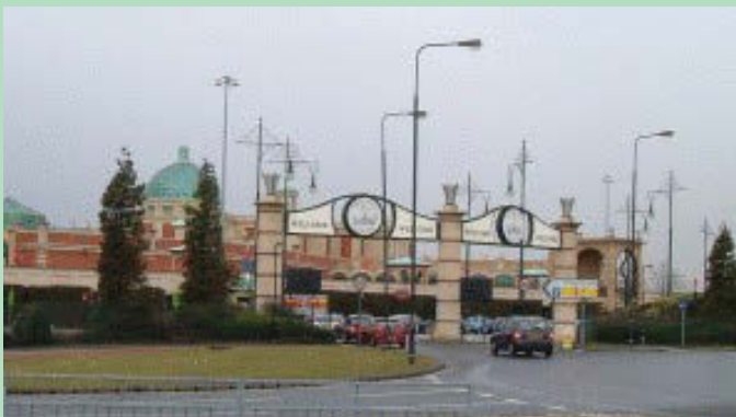
Picture 5.5 Trafford Centre
