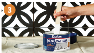
Add the additive and mix together
