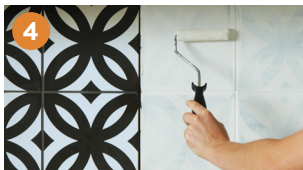
Roll on primer, topcoat and then clear coat
