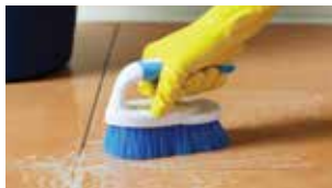
Scrub tiles before applying primer
