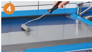
Roll on primer, topcoat and then clear coat
