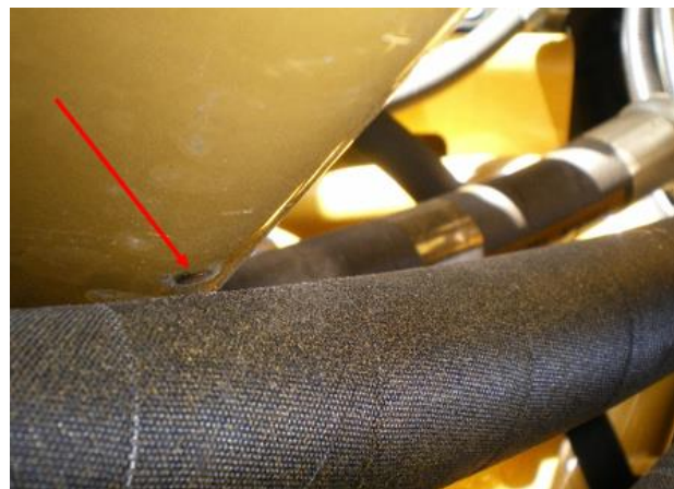
Figure 2. Chafe point on accessory drive shaft guard.
