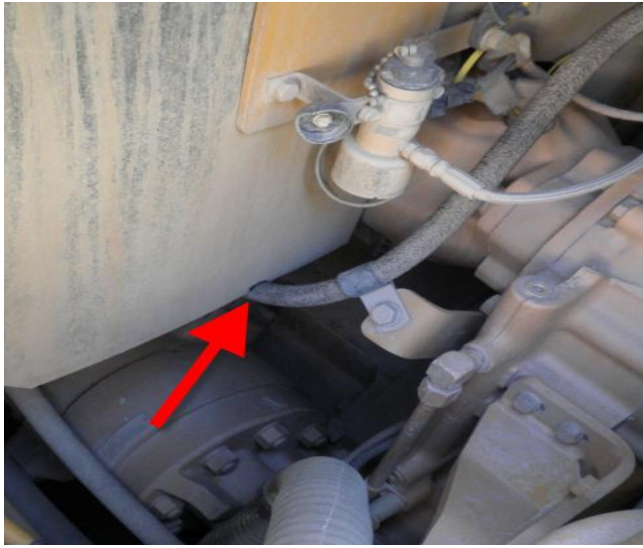
Figure 1 example of poorly routed fuel line.
