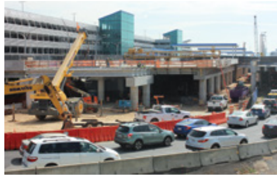
Elevated Roadway and Terminal Curb Front
