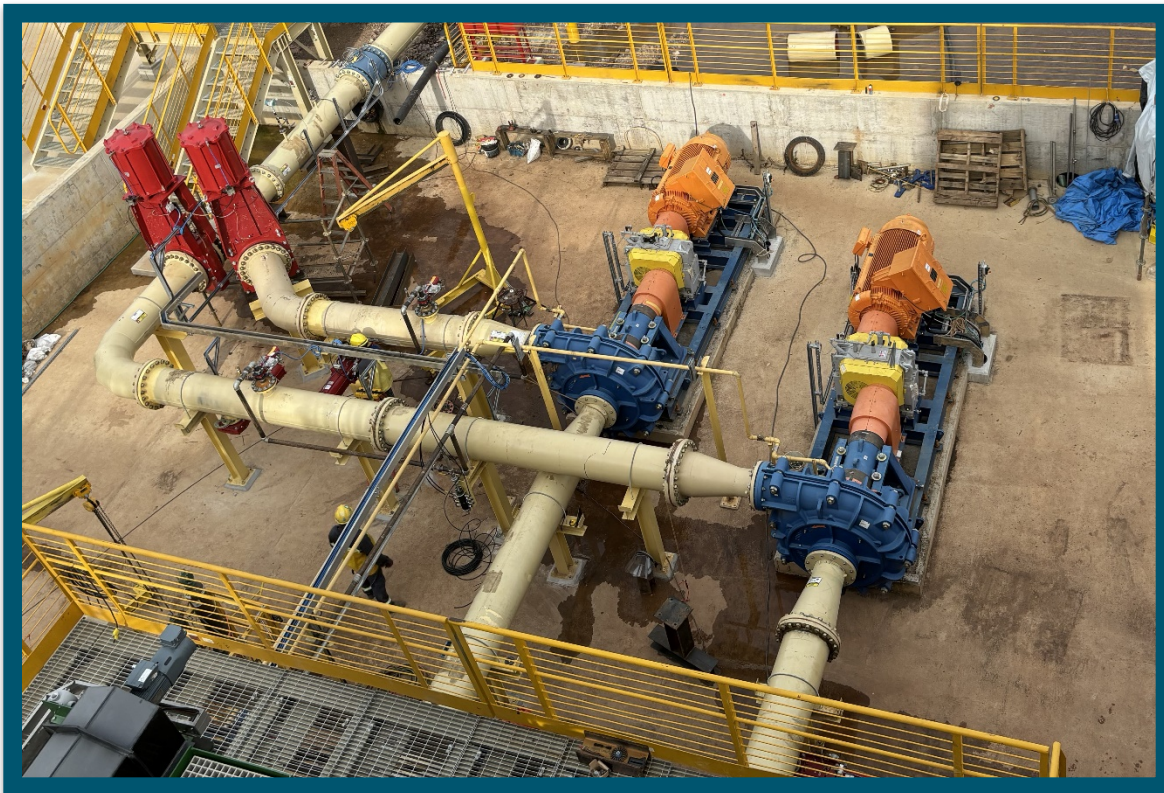
Figure 9 - Tailings Pumps
