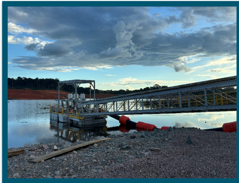
Figure 8 - Reclaim Barge
