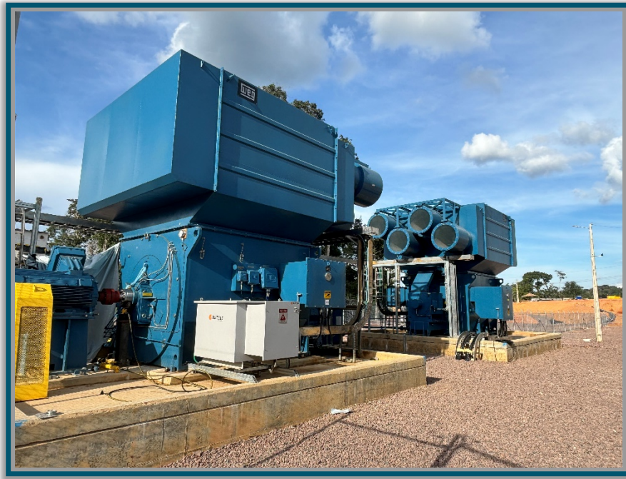
Figure 10 – Synchronous Condensers
