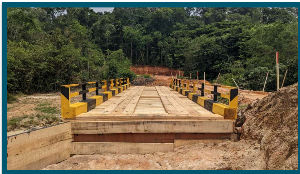
Figure 8 - Bridge Crossing Mine Access Road
