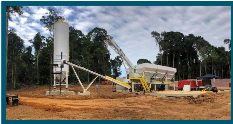
Figure 6 – Concrete Batch Plant Construction
