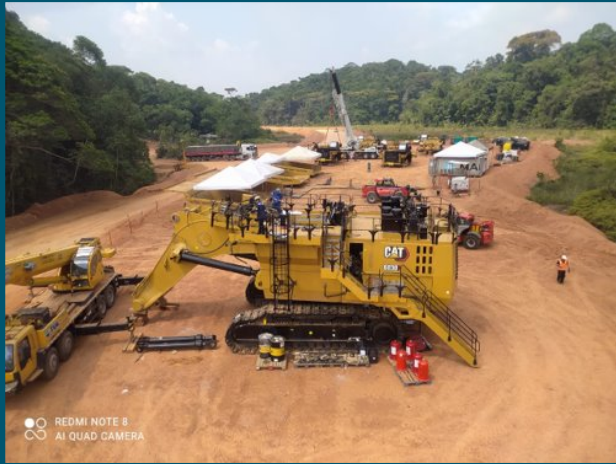
Equipment assembly pad
