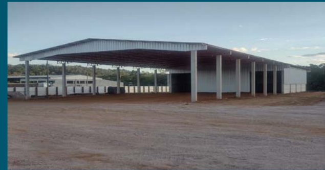
Morais Almeida Logistics Base Complete and Operational
