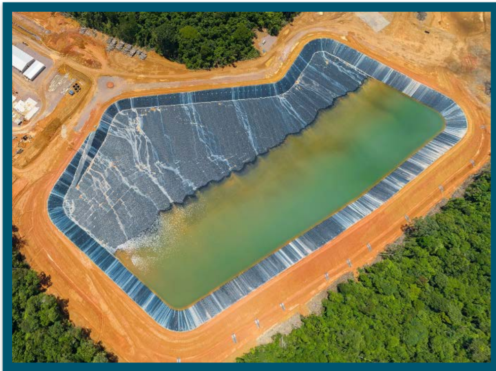
Figure 4 - CIL Tailings Storage Facility
