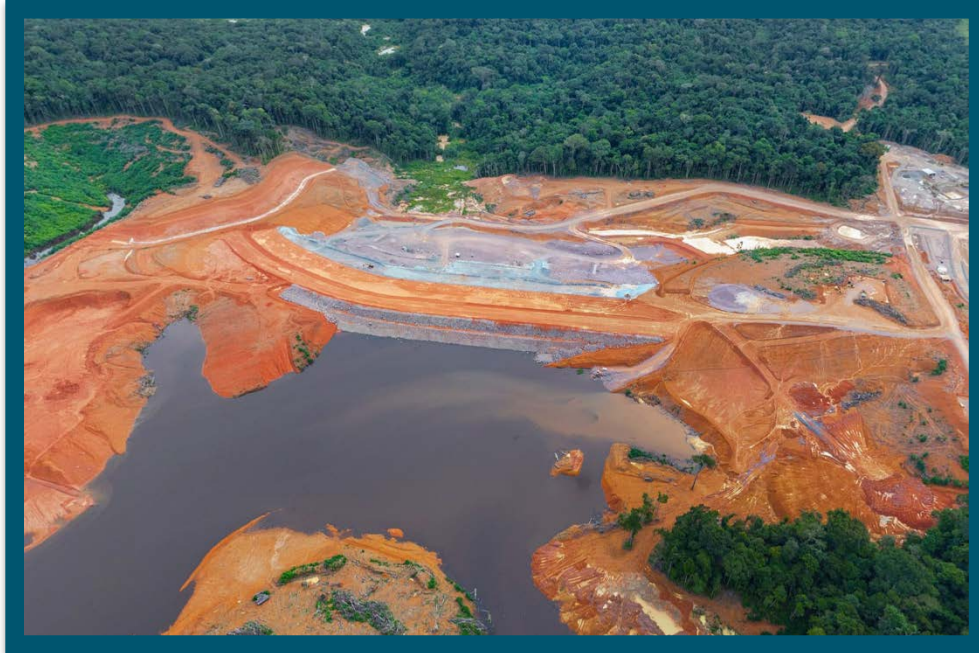
Figure 3 - Flotation Tailings Storage Facility
