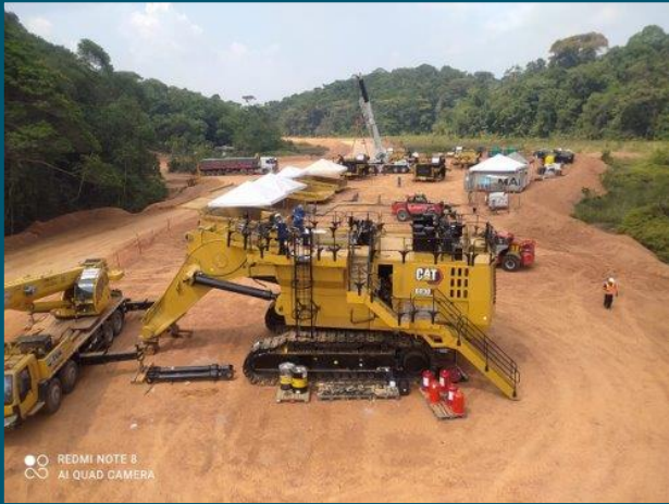
Equipment assembly pad
