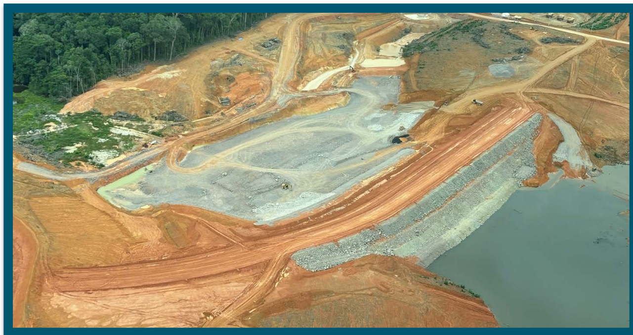
Figure 7 – Flotation Tailings Facility Main Dam
