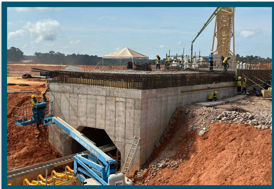
Figure 6 - Ore Reclaim Tunnel
