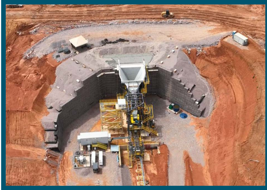
Figure 5 - MSE Wall & Primary Crusher
