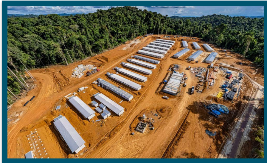
Figure 5 – Permanent Camp Construction
