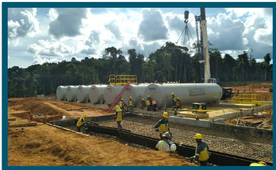
Figure 6 – Fuel Storage Tank Installation
