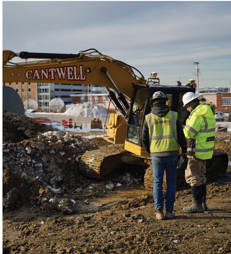
A common goal on a site is to have the project done on time and on budget - for every project.
