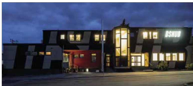
Drees & Sommer's Innovation Hub in Stuttgart, Germany is one of the locations where the company's employees cooperate with startups, clients, business partners or in collaborative research projects. © Peter Neusser
