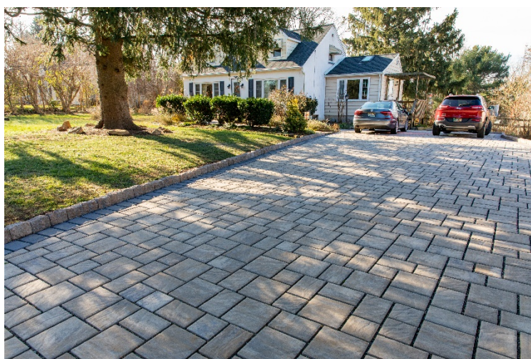
CO 2 -cured Solidia Concrete™ pavers installed in N.J., USA
