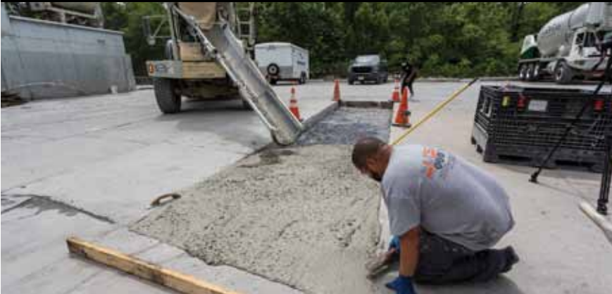
Figure 4: a demonstration pour of concrete with 20% Solidia SCM replacement for OPC
