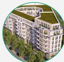
Elsenheimer Straße München-Sendling Housing units: ca. 350 Volume: 73 Mio. EUR
